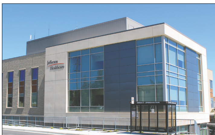
Jefferson Healthcare as viewed from Sheridan Street in Port Townsend. Courtesy of Jefferson Healthcare.
